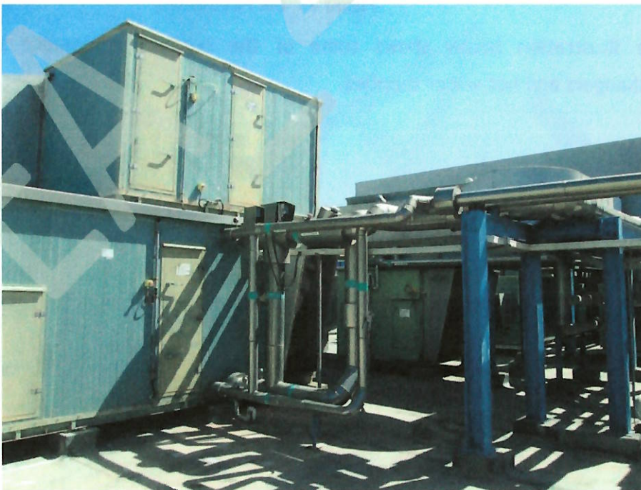
Figure 47. Air Handling Units
