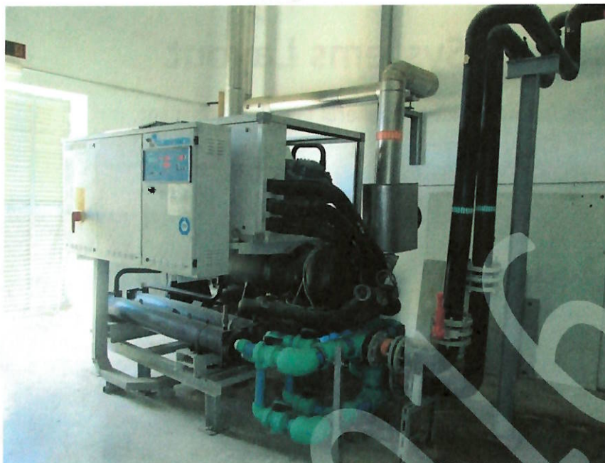
Figure 31. Chiller System_Small (Used as part of process)
