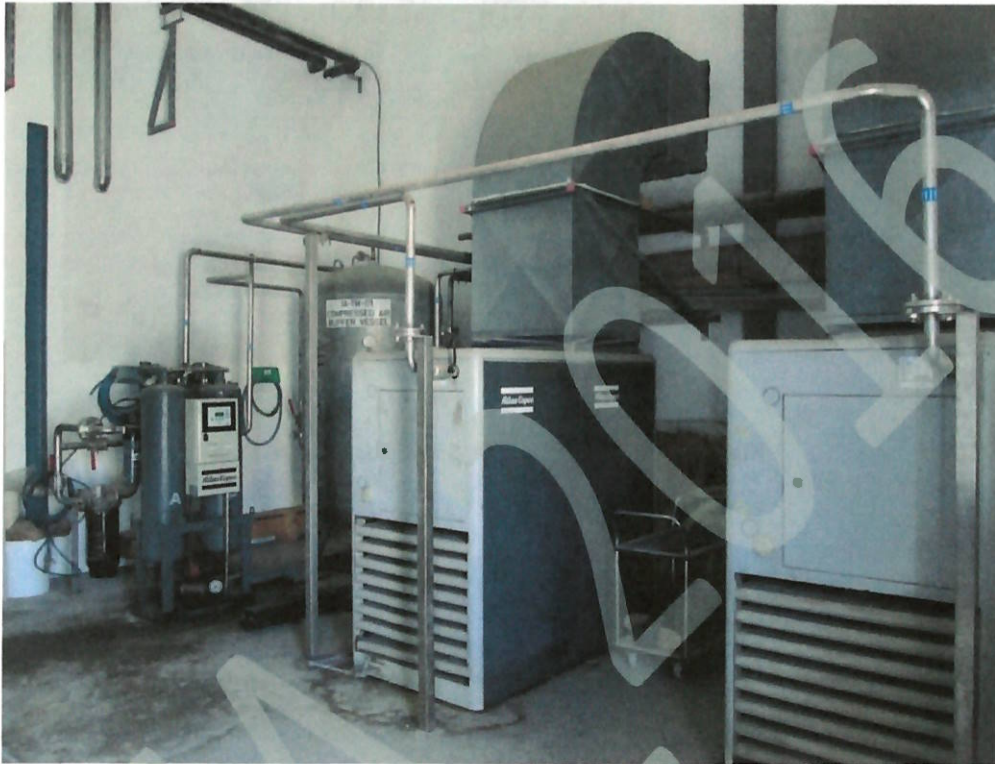
Figure 30. Air Compressors
