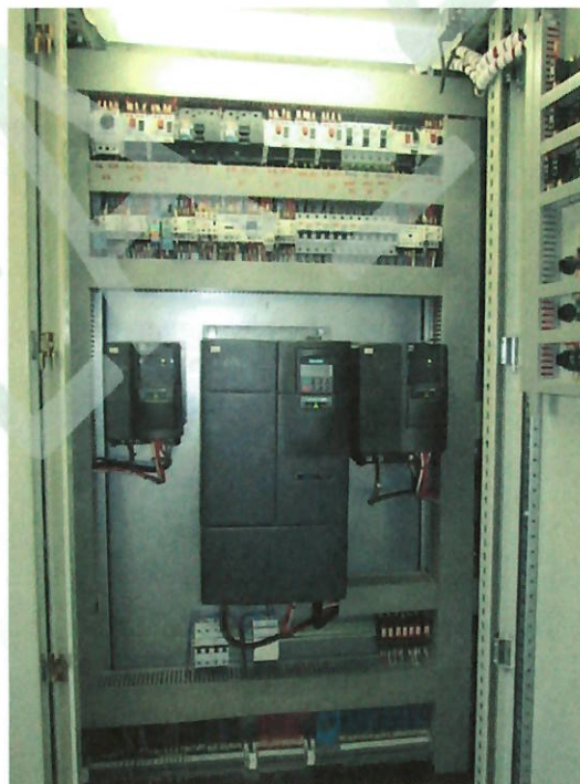
Figure 39. Variable Drive Unit_AHU
